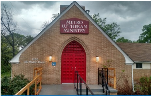
A new facility for Metro Lutheran Ministries' Northland operation, at St. James Lutheran
